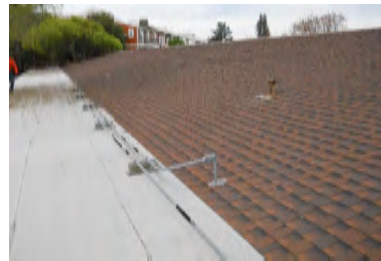
Roof Overview - Building 4
