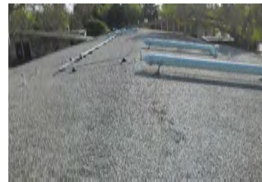
Roof Overview - Building 8
