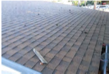
Roof Overview - Building 1
