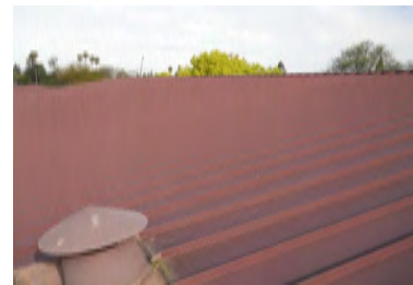
Roof Overview - Building B
