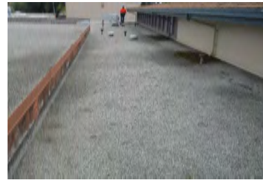
Roof Overview - Building 12
