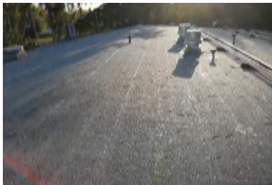
Roof Overview - Building 7
