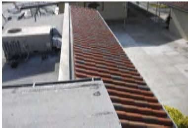
Roof Overview - Building 7A
