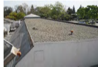
Roof Overview - Building 1100
