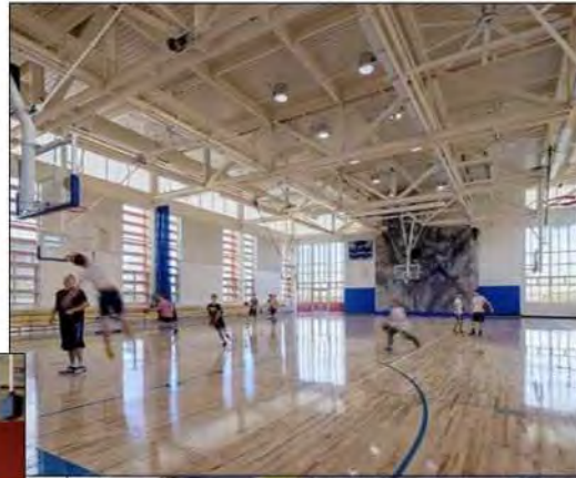
Upper Level Gym with Extensive Daylighting
