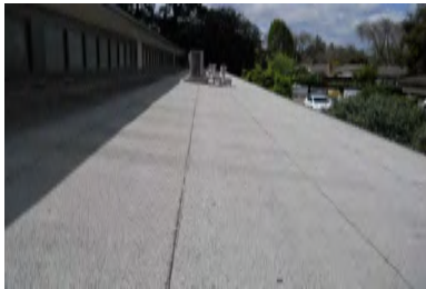
Roof Overview - Building 3 (Building 4&5 Similar)
