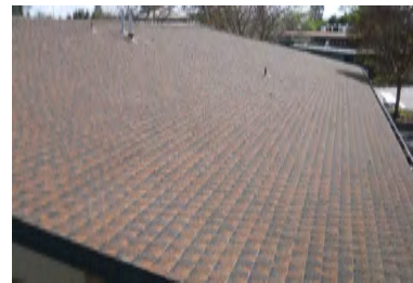
Roof Overview - Building 5 (Buildings 6 Similar)
