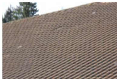
Roof Overview - Building 1100
