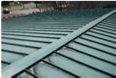
Roof Overview - Building E
