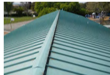
Roof Overview - Building N
