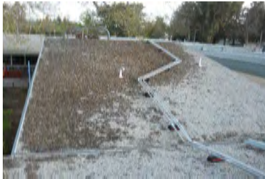
Roof Overview - Building Admin. Office
