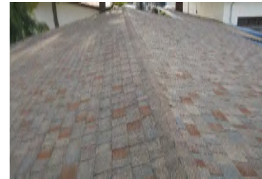
Roof Overview - Building 100
