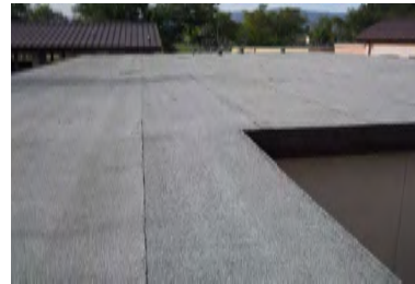
Roof Overview - Building F
