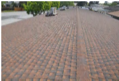
Roof Overview - Building 11
