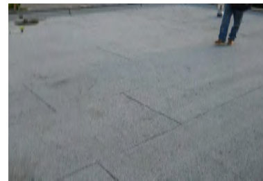
Roof Overview - Building 2 (Building 3 Similar)
