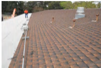
Roof Overview - Building 5
