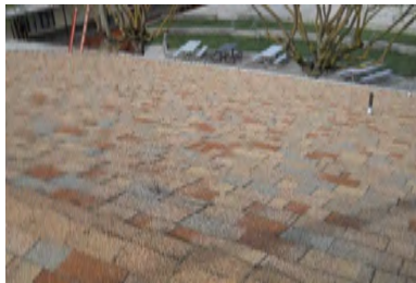
Roof Overview - Building 800
