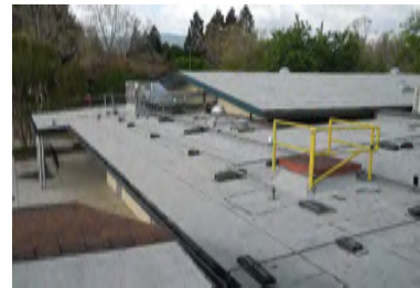
Roof Overview - Building 9
