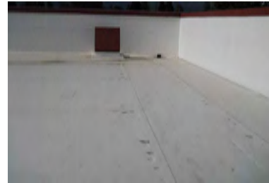
Roof Overview - Building 7B
