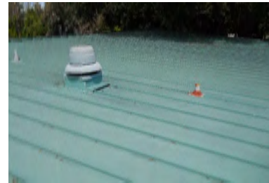
Roof Overview - Building C
