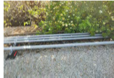
Typical Deficiency - Debris have accumulated at field of roof. Recommend trimming trees back from roof eaves, clearing debris from all gutters, drains, waterways, and field of roof to promote positive drainage.
