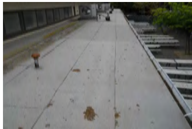
Roof Overview - Building 5
