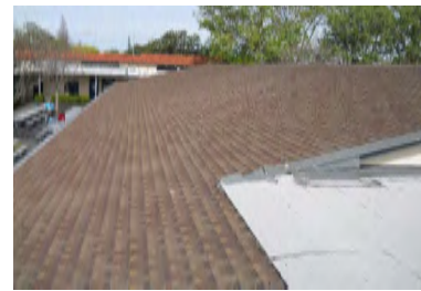
Roof Overview - Building K
