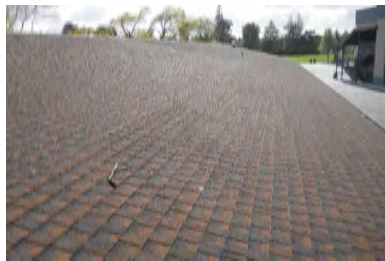
Roof Overview - Building 2 (Buildings 3, 4, and 8 Similar)
