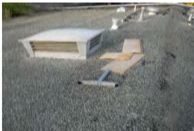
Roof Overview - Building 5
