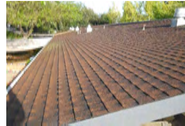
Roof Overview - Building 5 and 6 Similar
