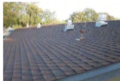
Roof Overview - Building 3
