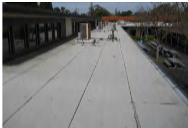
Roof Overview - Building L
