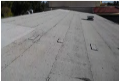
Roof Overview - Building 7A
