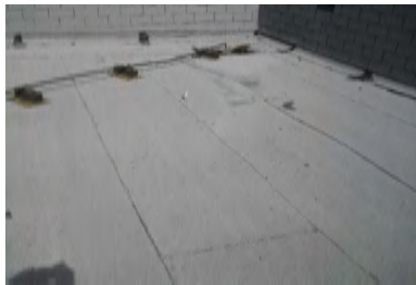
Roof Overview - Building P
