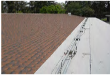
Roof Overview - Building 1&2
