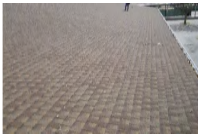
Roof Overview - Building J
