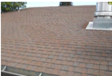
Roof Overview - Building 2
