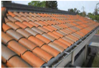
Roof Overview - Building P
