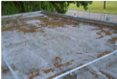
Roof Overview - Building 1
