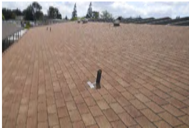
Roof Overview - Building 13
