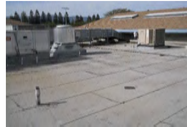
Roof Overview - Building 800
