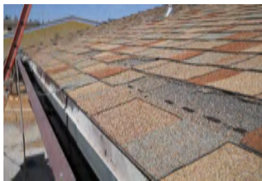
Typical Deficiency - Asphalt shingles are damaged and missing. Recommend replacing as needed.
