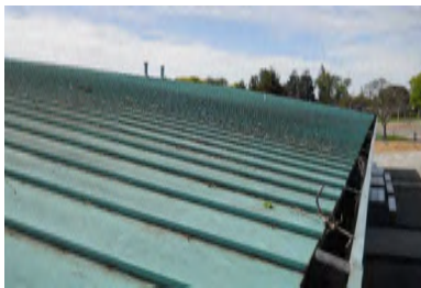
Roof Overview - Building P
