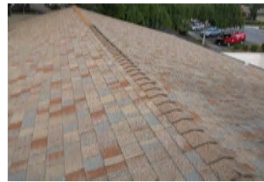
Roof Overview - Building 700
