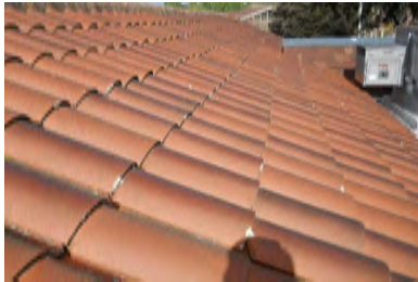
Roof Overview - Building 1
